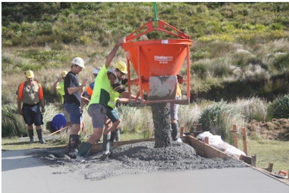
Kibble on 30m long line from helicopter
