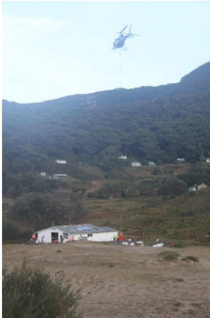
Kibble on 30m long line from helicopter
